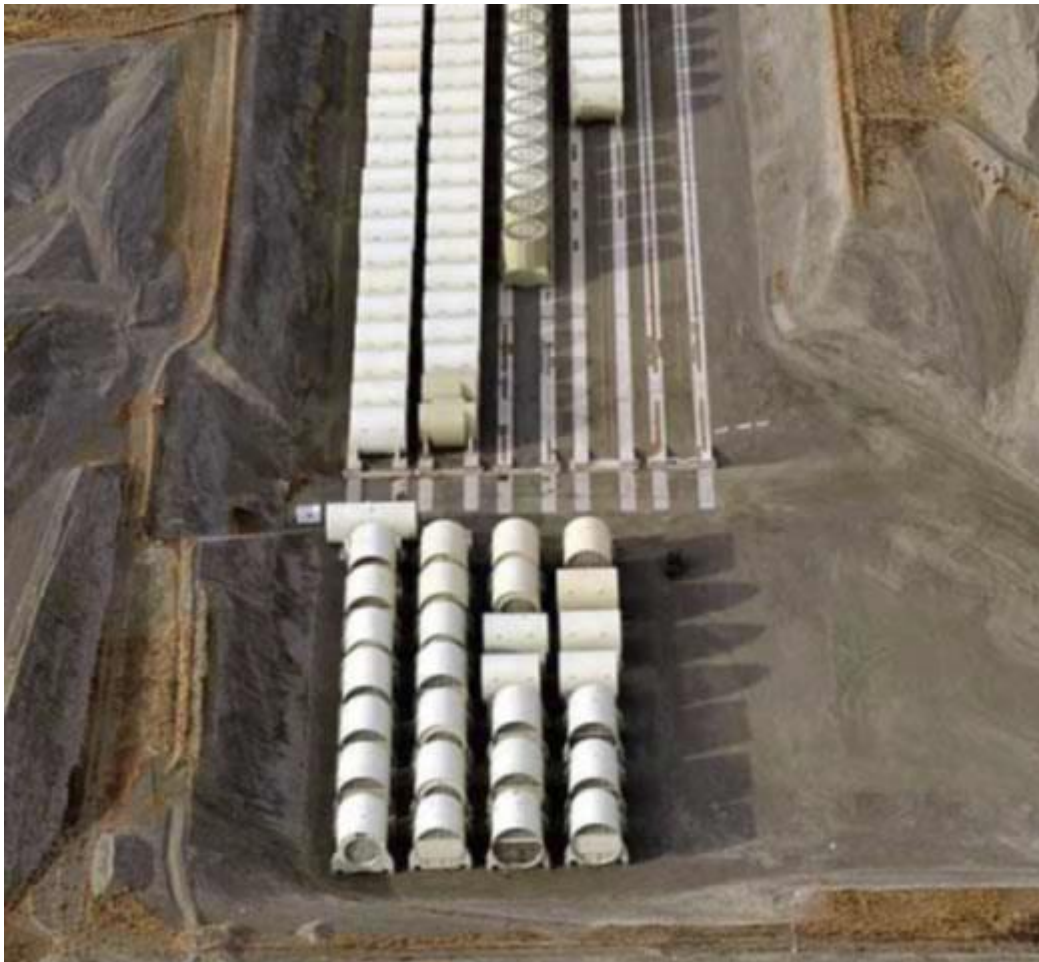
Left : A disposal site with reactors from cruisers and Los Angeles-class subs in Hanford,
